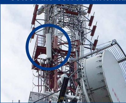
Access roof or tower and select the antenna you want to align.
